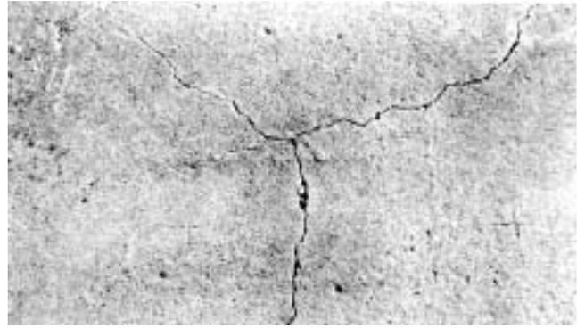
Fig. 11.1—Drying-shrinkage cracks such as these are a frequent cause of complaint (PCA A5271).
