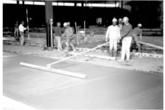
Fig. 8.6—“Modified highway” straightedge.
