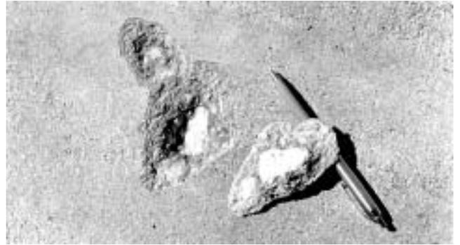
Fig. 11.7—A popout is a small fragment of concrete broken away from the surface of a slab due to internal pressure, leaving a shallow, typically conical, depression (PCA 0113).
