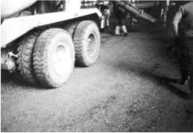
Fig. 4.1—Proof-rolling by loaded ready mix truck.
