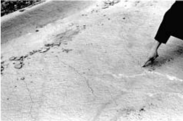
Fig. 11.2—Plastic-shrinkage cracks are caused by rapid loss of mixing water from the surface while the concrete is still plastic (PCA 1311).
