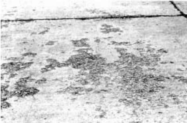
Fig. 11.5—Scaling is the loss of surface mortar, usually exposing the coarse aggregate (PCA A5273).
