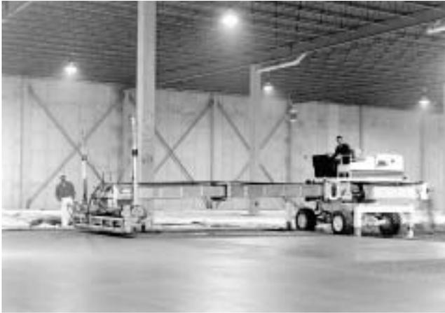
Fig. 8.4—Laser-controlled screed.
