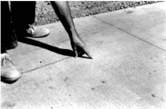
Fig. 11.3—Crazing is a network of very fine superficial surface cracks (PCA 4099).
