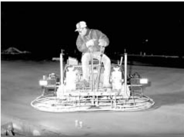
Fig. 8.5—Double-riding trowel with clip-on pans.
