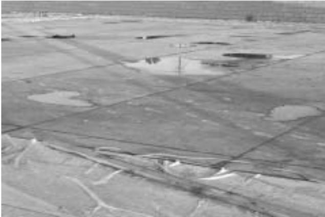
Fig. 11.11—Low spots in a slab after rain shower (courtesy of Eldon Tipping).
